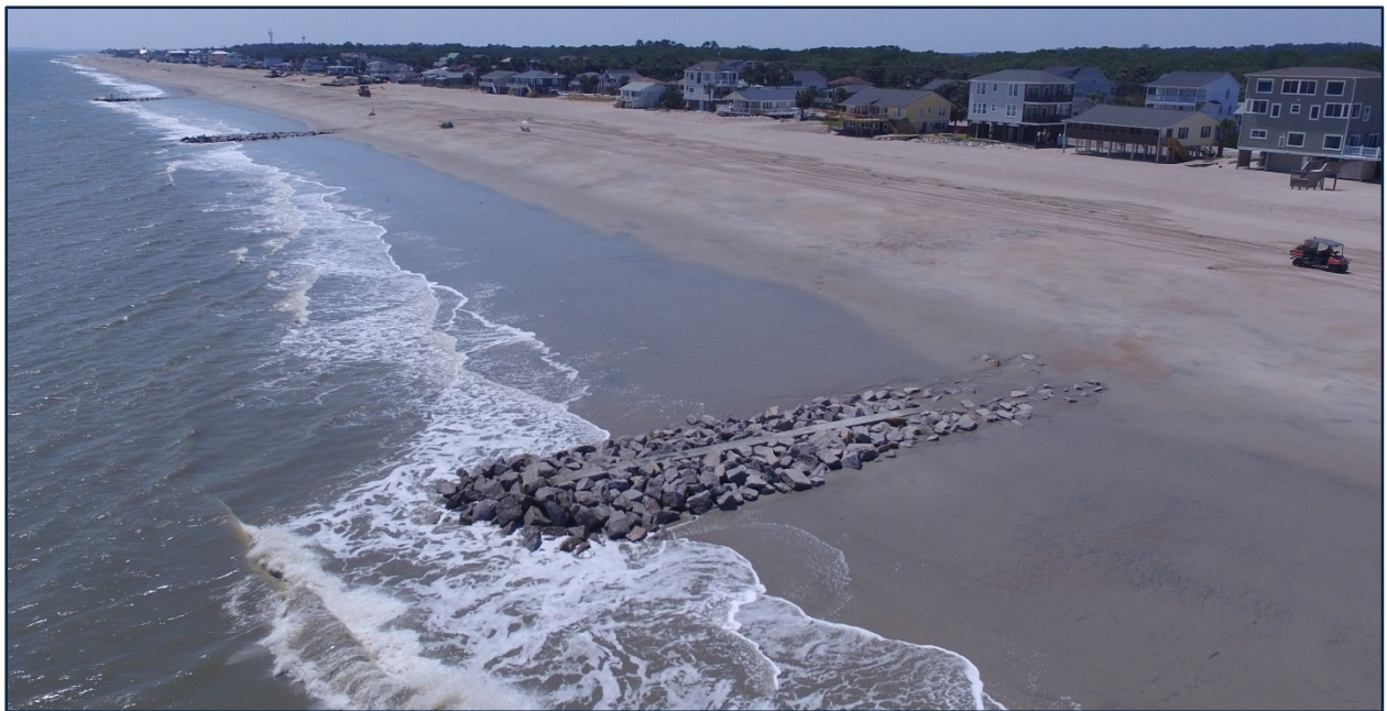
FIGURE 3.10. [UPPER] Pouring concrete cap on the landward end of groin extension. [LOWER] Completed extensions for Groin 7 (foreground), Groin 8 (middle), and Groin 9 (background).
