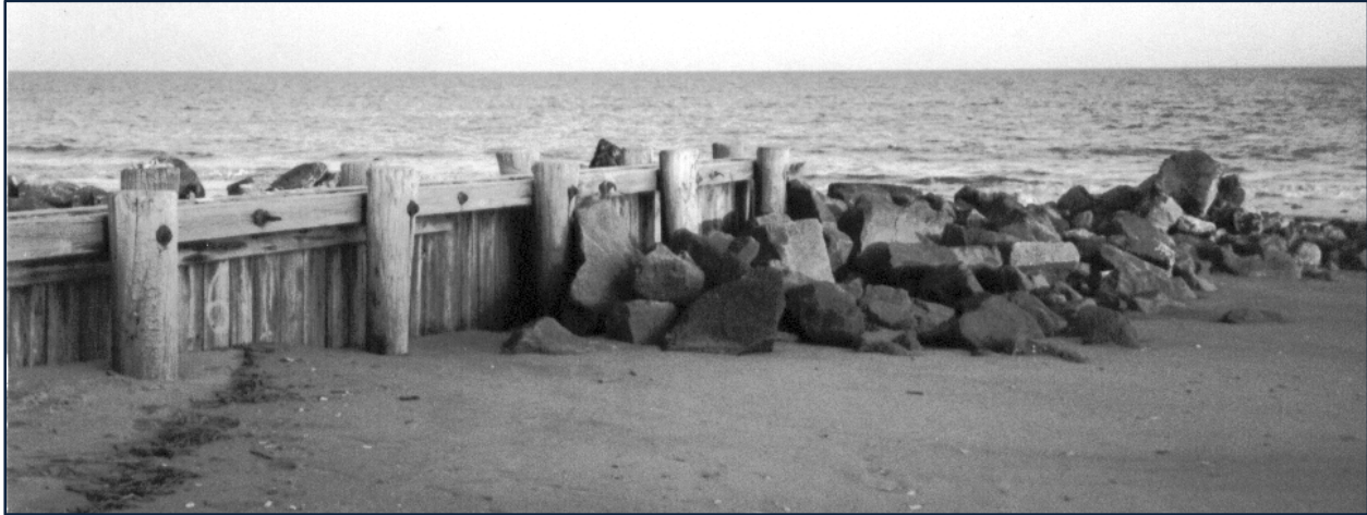
FIGURE 2.4. Typical Edisto Beach (SC) groin prior to the 1995 repair project.
