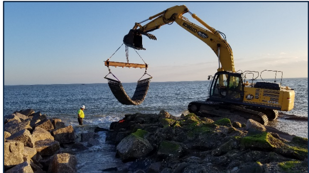
FIGURE 3.7 Images of the groin construction.
