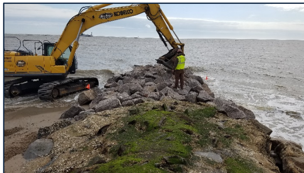
FIGURE 3.7 Images of the groin construction.
