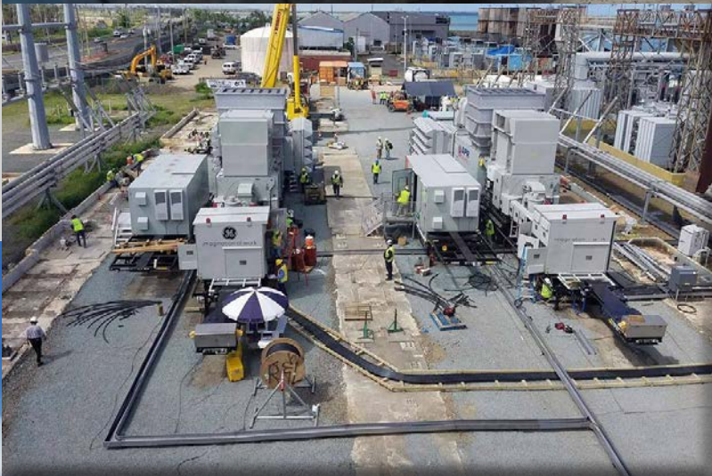
Opposite Left: Ryan Bamberg, Charleston District, and Dustin Tellinghuisen, Buffalo District, take notes while they complete their assessment of a building in Puerto Rico. Opposite Right: Matt Boles surveys Folly Beach to determine how much sand was lost during Hurricane Irma. Top: Brig. Gen. Diana Holland South Atlantic Division Commander, surveys Guajataca Dam, Puerto Rico. Middle Left: U.S. Army Corps of Engineers Task Force Power Restoration Team works to install two generators at a power plant in Puerto Rico. Middle Right: An aerial view of blue roofs on homes provided by the U.S. Army Corps of Engineers. Bottom: Contractors working for the U.S. Army Corps of Engineers install a temporary blue roof in Puerto Rico.
