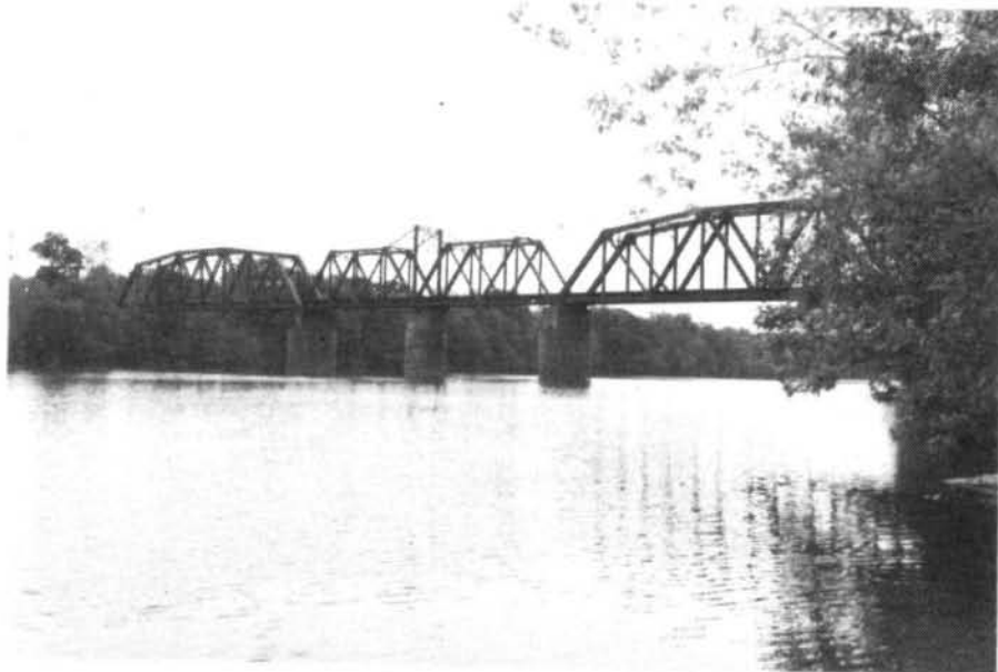
FIGURE 4 - SEABOARD COAST LINE RAILROAD BRIDGE (R.M. 36.3)
