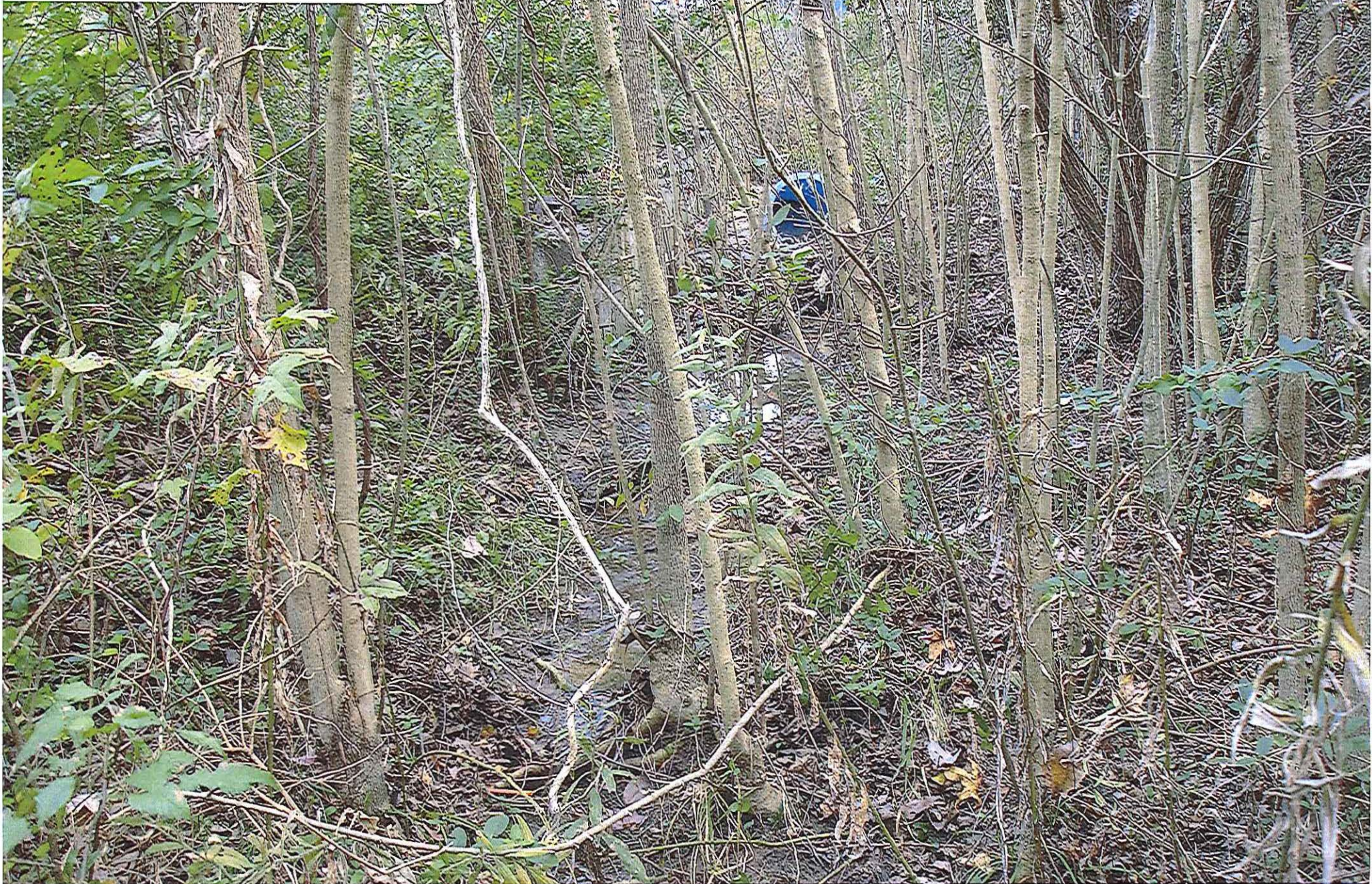
Photo 3 SCDOT US 21 & SC-51, York Co Wetland D. Photo taken 11/17/15 facing east in drainage way below retaining walls adjacent to 24" culvert under US 21
