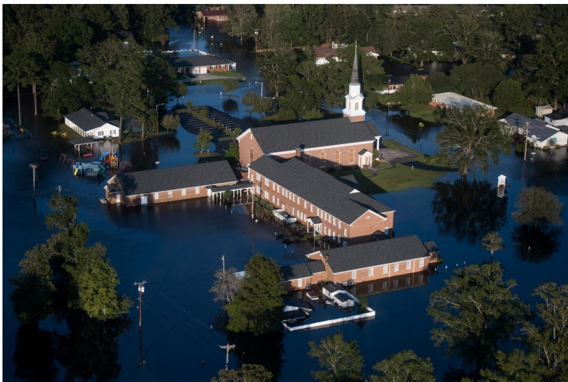
Figure B-10. Flooding from Hurricane Florence, 2018 in Conway, SC (Horry County, 2021)
