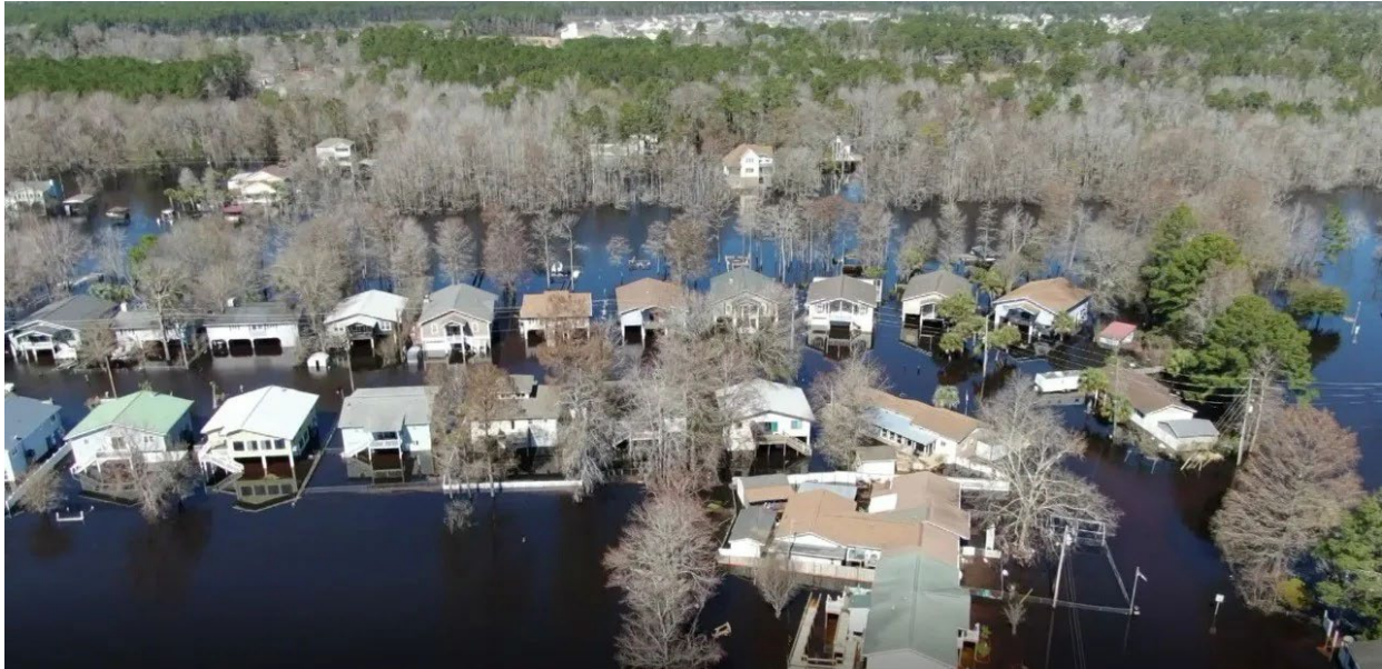
Figure B-19. Flooded Homes and properties in Socastee during Hurricane Florence (Horry County (2021))
