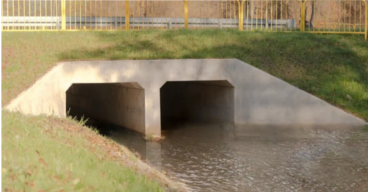
Figure B-1: Box Culvert with Wingwalls example
