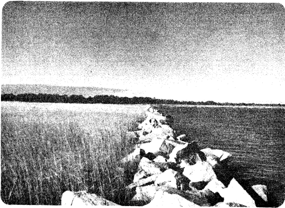
Plate 2B. Low marsh, left, formed after rock jetty was constructed at the mouth of Winyah Bay, right. Oak-pine forest is seen in background on South Island.
