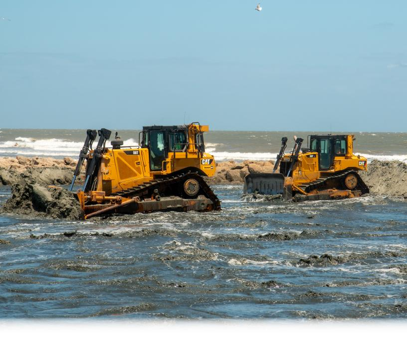
wide dune extending from the southern end of the state park southward for over 16,000 feet past the southern point of the island. The dune will be fronted by a berm of varying widths. The project also includes lengthening select groins along the beach front.
