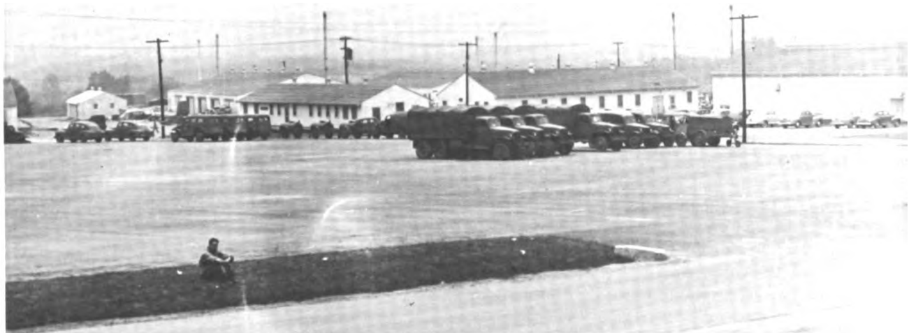
Construction at Charleston Air Force Base during the Korean War, barracks and the chapel.
