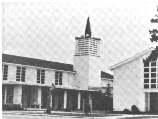
Construction at Charleston Air Force Base during the Korean War, barracks and the chapel.
