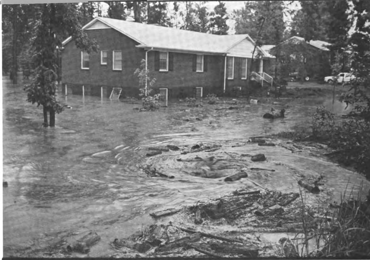
Flood control. Flooding in the tributary to Briar Creek in 1964; Small Flood Control project under construction near Summerville, South Carolina.
