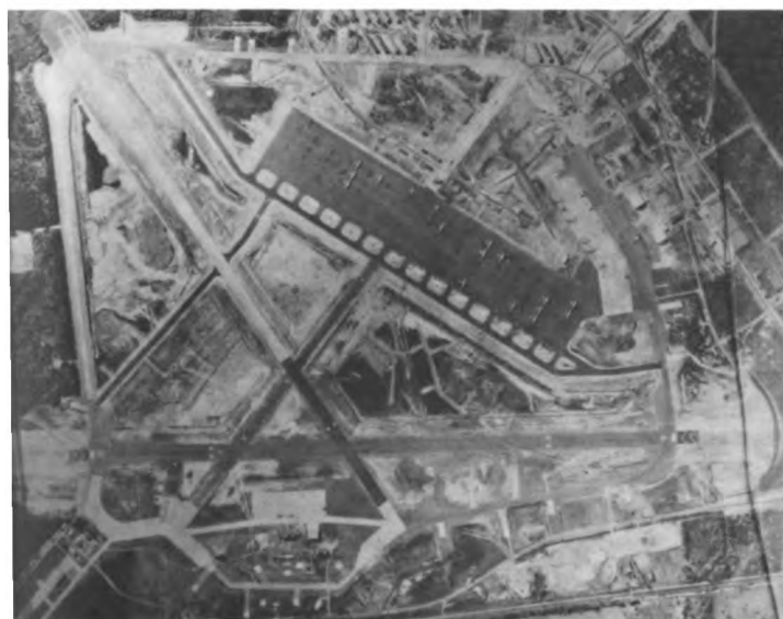
Charleston airport construction, World War II and enlargement during the Korean War.
