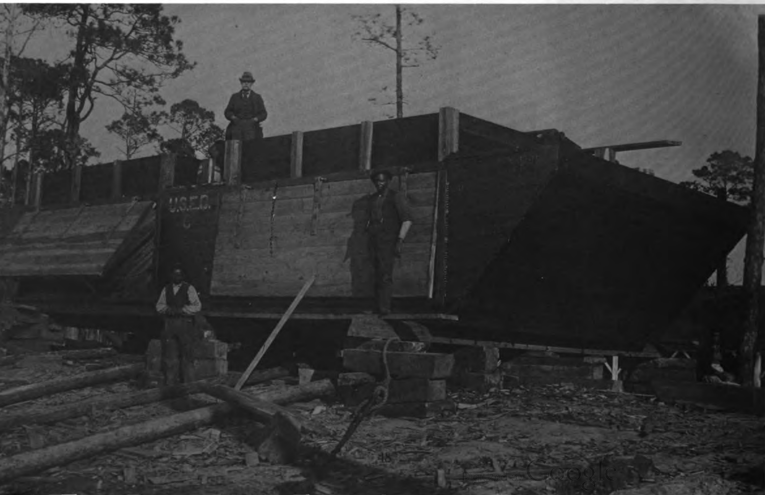
Work on the Santee River in 1895. The dump scow C , built at the Corps of Engineers saw mill, for use on the Estherville and Minim Creek Canal.
