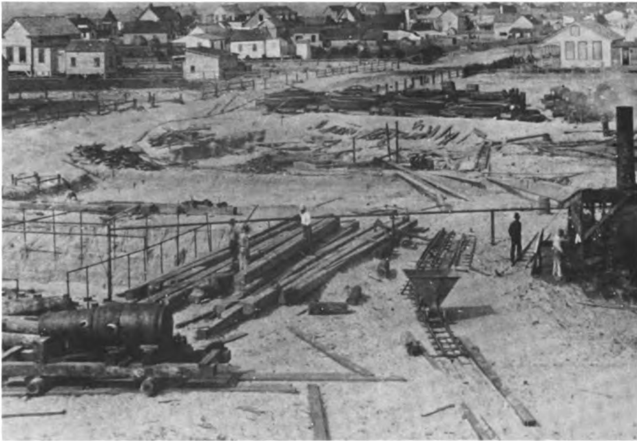
Construction scenes. Fort Moultrie and Battery Jasper, 1897-1898.
