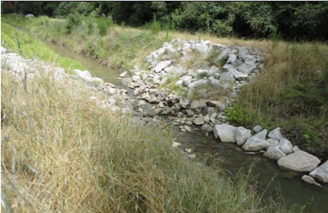
**Figure 6. Low-head Rock Weirs Designed by NRCS.**
