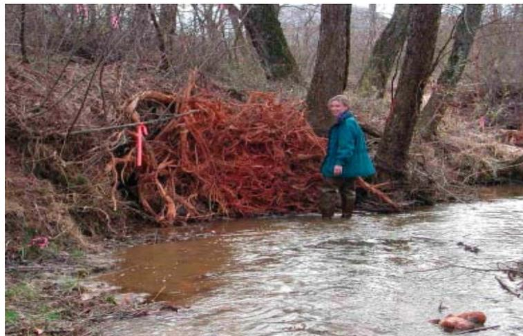
**Figure 13. An example of Root Wads Placed along a Stream Bank to Improve Newberry Rock Riffle Morphologic Heterogeneity.**
