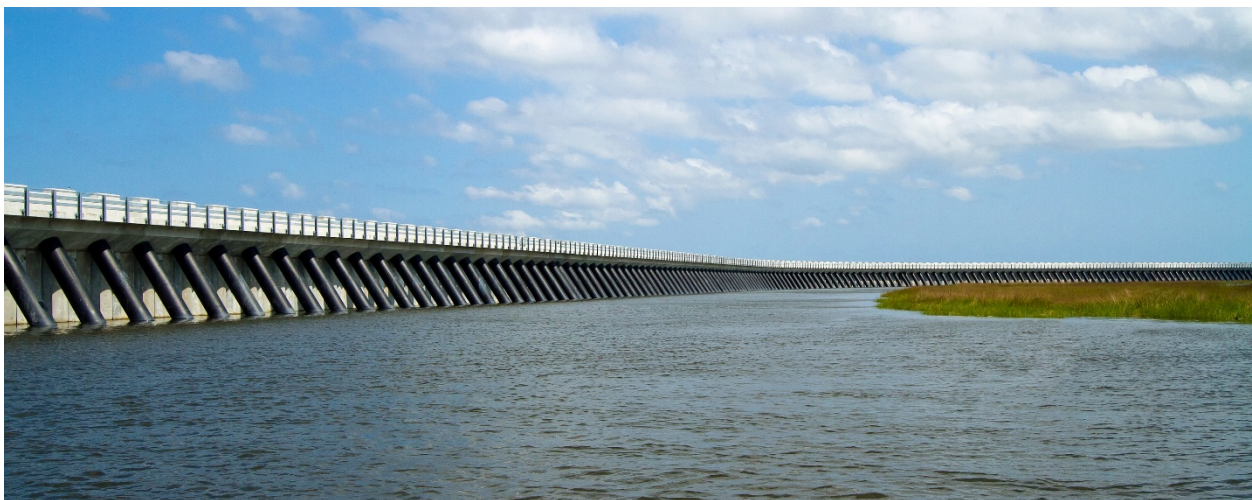
Figure 3-4. The Inner Harbor Navigation Canal Surge Barrier in New Orleans is an example of an approximately 26 feet (NAVD88) combo-wall.
