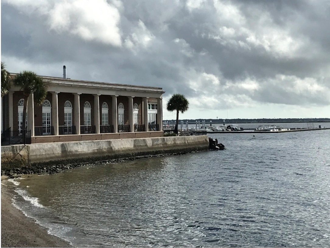
Figure 4-11. Seawall by the Carolina Yacht Club along the Charleston Harbor. It is reinforced at the toe with rip rap. Rip rap continues around the corner along the east side of the yacht club (out of view in this photo)
