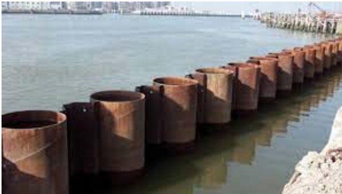
View of Constructed Combo Wall Substructure
