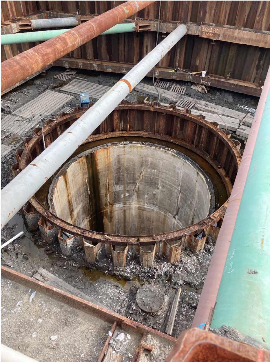
150' deep wet well shaft in shored excavation
