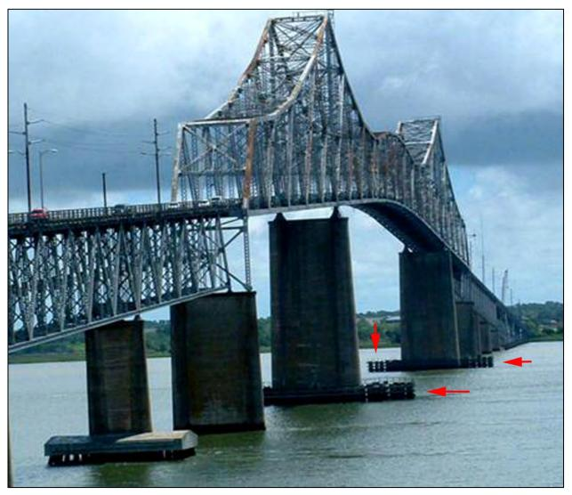
Figure 49. Bridge bent cribbing on the John P. Grace Bridge. A section from this bridge is thought to represent the wooden object noted in the acoustic image (photo by Sharon Bohn courtesy of <a href="https://www.notablephotos.com">www.notablephotos.com</a>).
