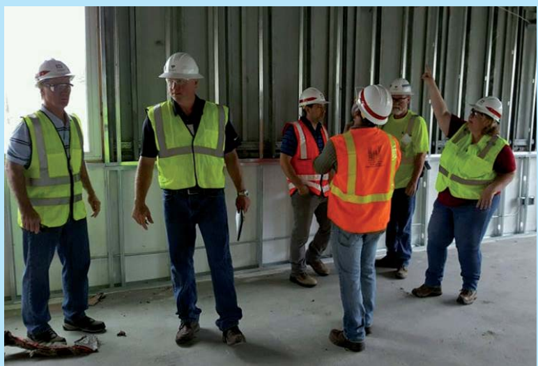
Top: Brandon Works, engineer, inspects the sub-floor.
